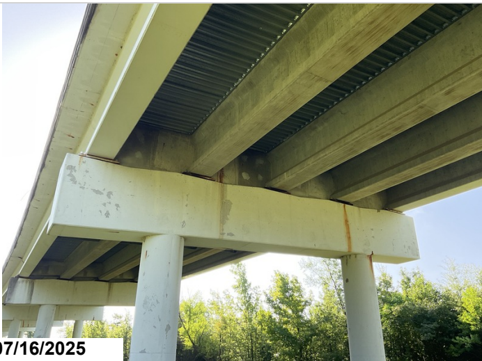
The bridge bearings are rated a 6 this inspection due to various bearings starting to rust.
