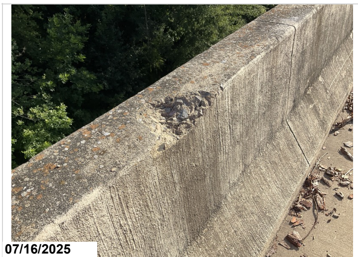
Left side, bridge railing, 1' of spalling, CS2.
