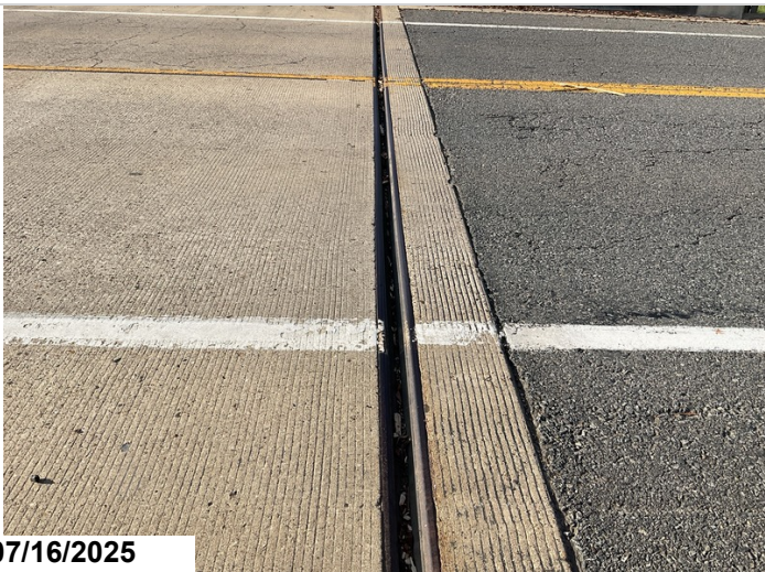
Bent 1 approach joint, debris impactation, CS2.
