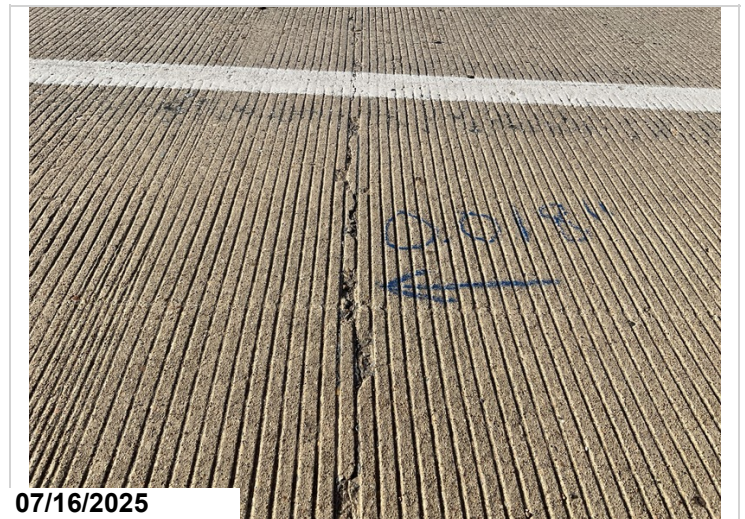
The approach spans and main spans have cracking in various locations throughout the topside of the deck.
