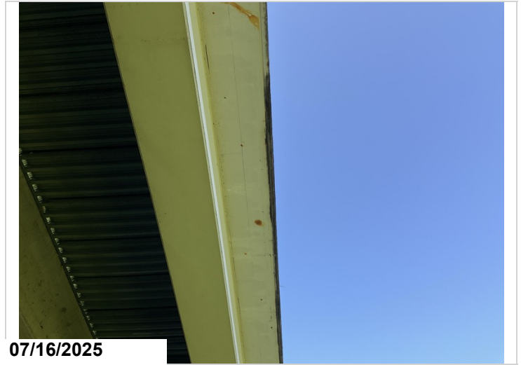
The left and right side concrete overhangs have cracking with efflorescence in various locations, CS2.
