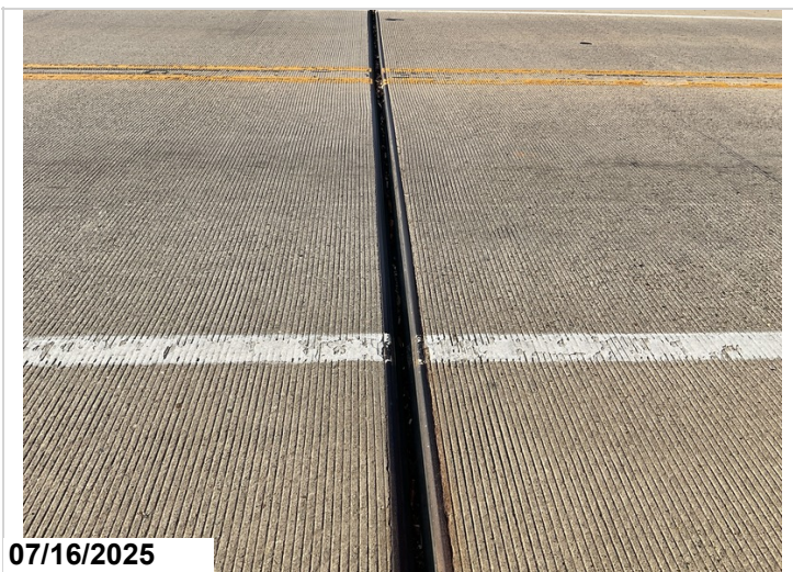
Bent 9 joint, main span, 30' of debris impaction, CS2.
