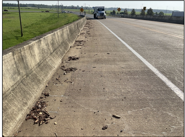
The left and right sides of the gutter lines have debris buildup. Note: The debris buildup is tree bark due to excessive amounts of large trucks.
