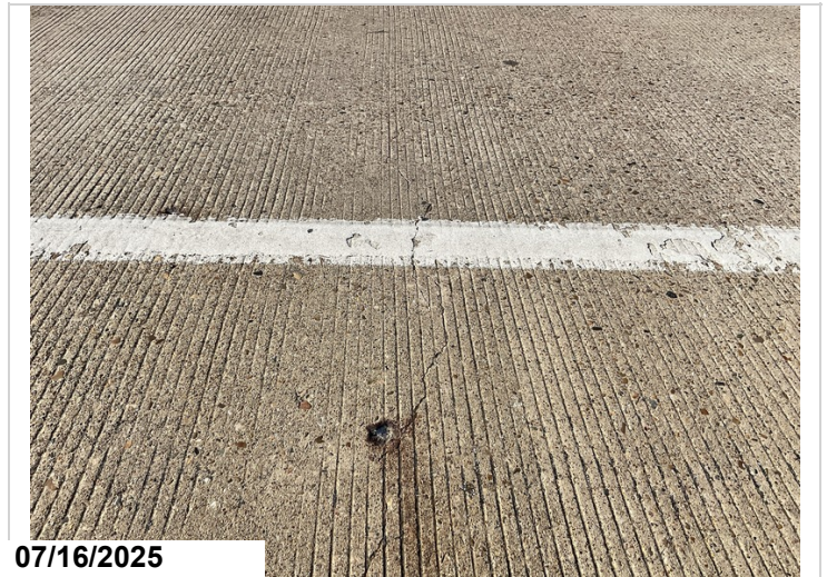
The approach slab has of cracking in various locations, CS2.
