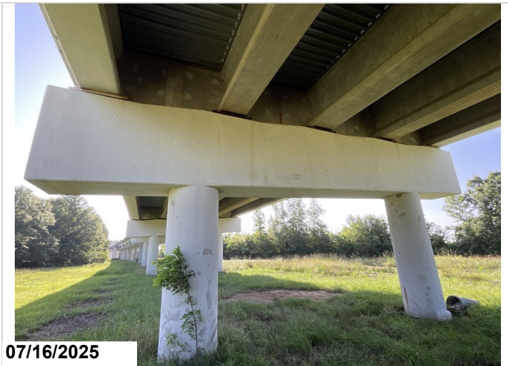
Typical photo of the concrete pier cap
