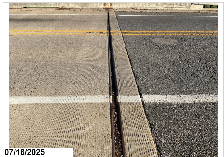
Bent 21 joint, approach span, debris impaction, CS2.
