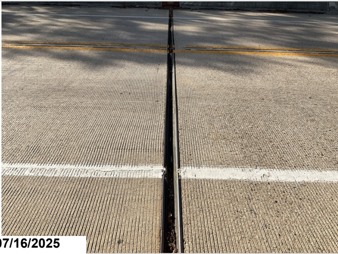
Bent 17 joint, approach span, debris impactation, CS2.
