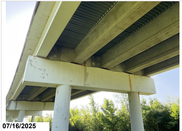
Various bearings are starting to rust, CS2.
