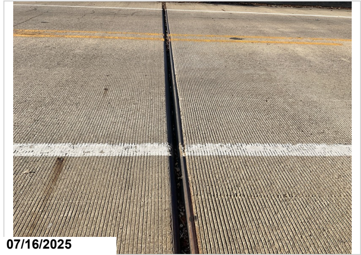
Bent 5 joint, approach slab, debris impactation, CS2.
