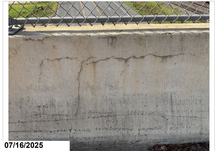
Concrete bridge railing, left and right sides, main spans, cracking in various locations, CS2.
