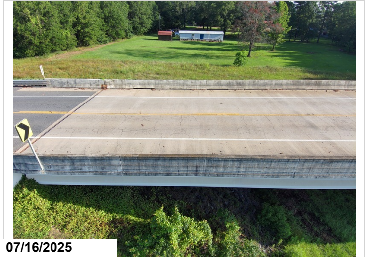
Cracks along the topside of the deck have been sealed.
