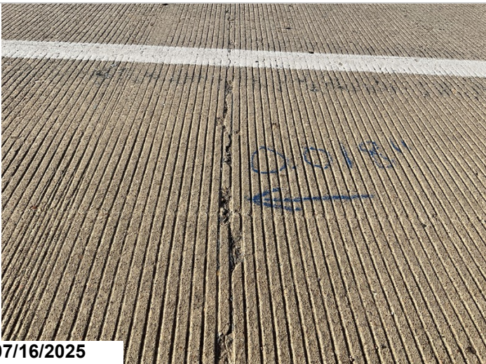
The approach slab has of cracking in various locations, CS2.
