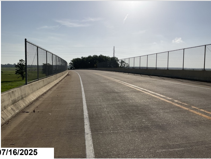
Fence is mounted to parapet wall.
