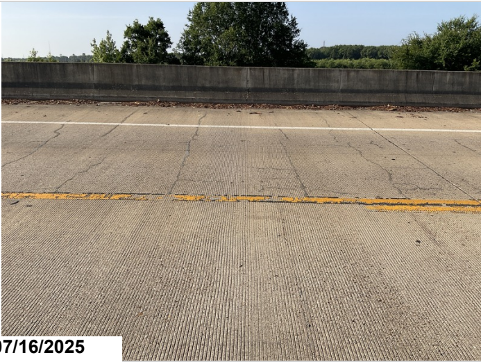
Various cracks along the main spans and approach spans have been sealed.
