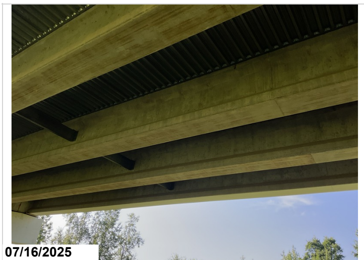
Typical photo of the prestressed concrete I-beams.
