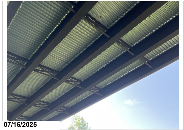
Typical photo of the weathering steel beams.
