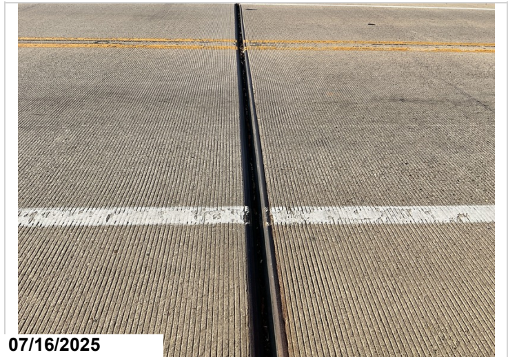
The bridge joints are rated a 6 this inspection due to there being debris impact in various locations.
