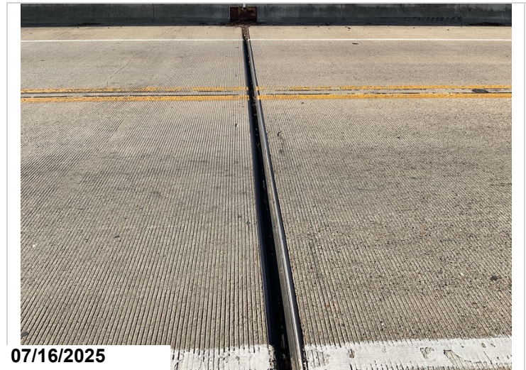
Bent 13 joints, main span, 30' of debris impaction, CS2.
